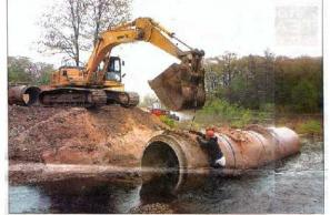
Seoff Gowin secures one of five 60-inch concrete pipes Thursday before it is removed from Ruddiman Grack. The pipes were put in to allow a continued flow of water during the 10 months of construction and cleanus
